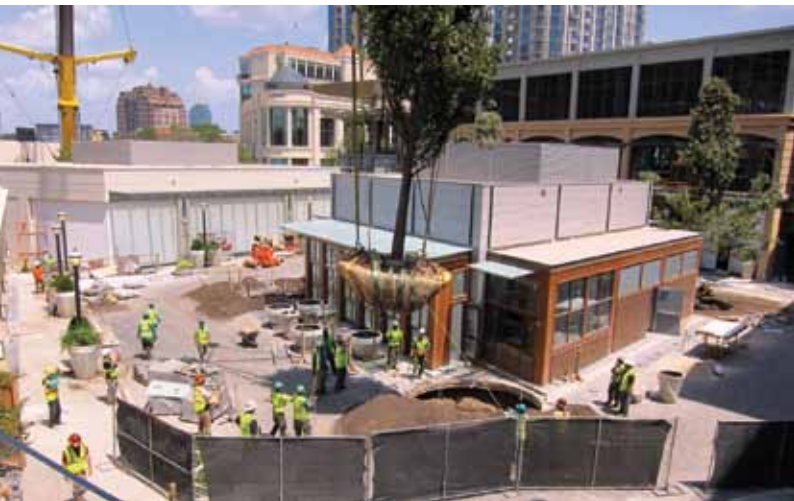
These 40' oaks, with their 13' diameter rootballs, were precisely guided into pre-finished 14' diameter holes using radio communication between ground personnel and the crane operator.
