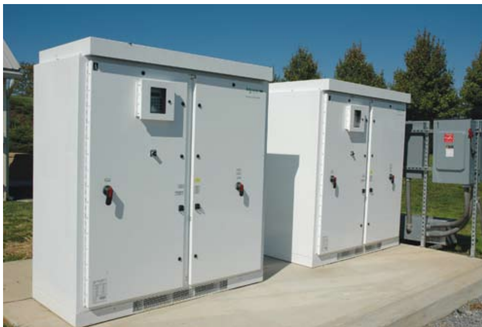
Solar panels consist of a series of photovoltaic cells that convert energy from the sun into direct current (DC). In order for that electricity to be used in a home or facility, it must be converted to alternating current (AC) using an inverter, pictured here.
